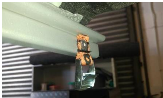
Figure 11: Buckle strap riveted onto awning arm
